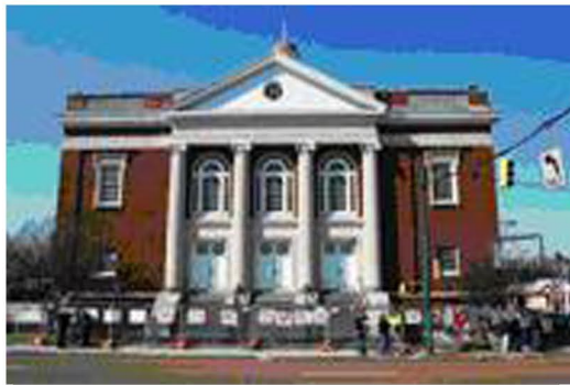
Union Ave. United Methodist Church, Memphis, TN Photo credit: James F. Williamson
